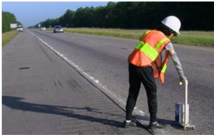
25 (b) Manually measure faulting on the roadway
