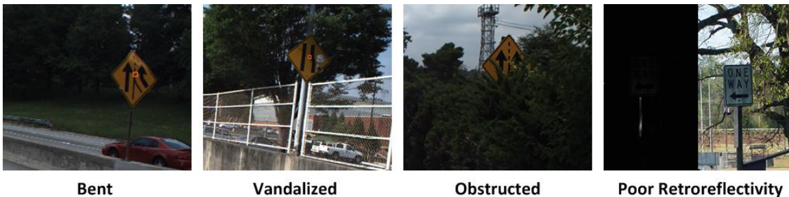
108 FIGURE 1 Typical traffic sign damages and poor conditions
